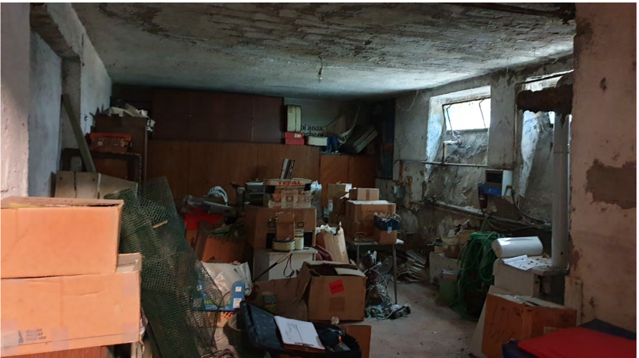
VISTA PIANO INTERRATO
