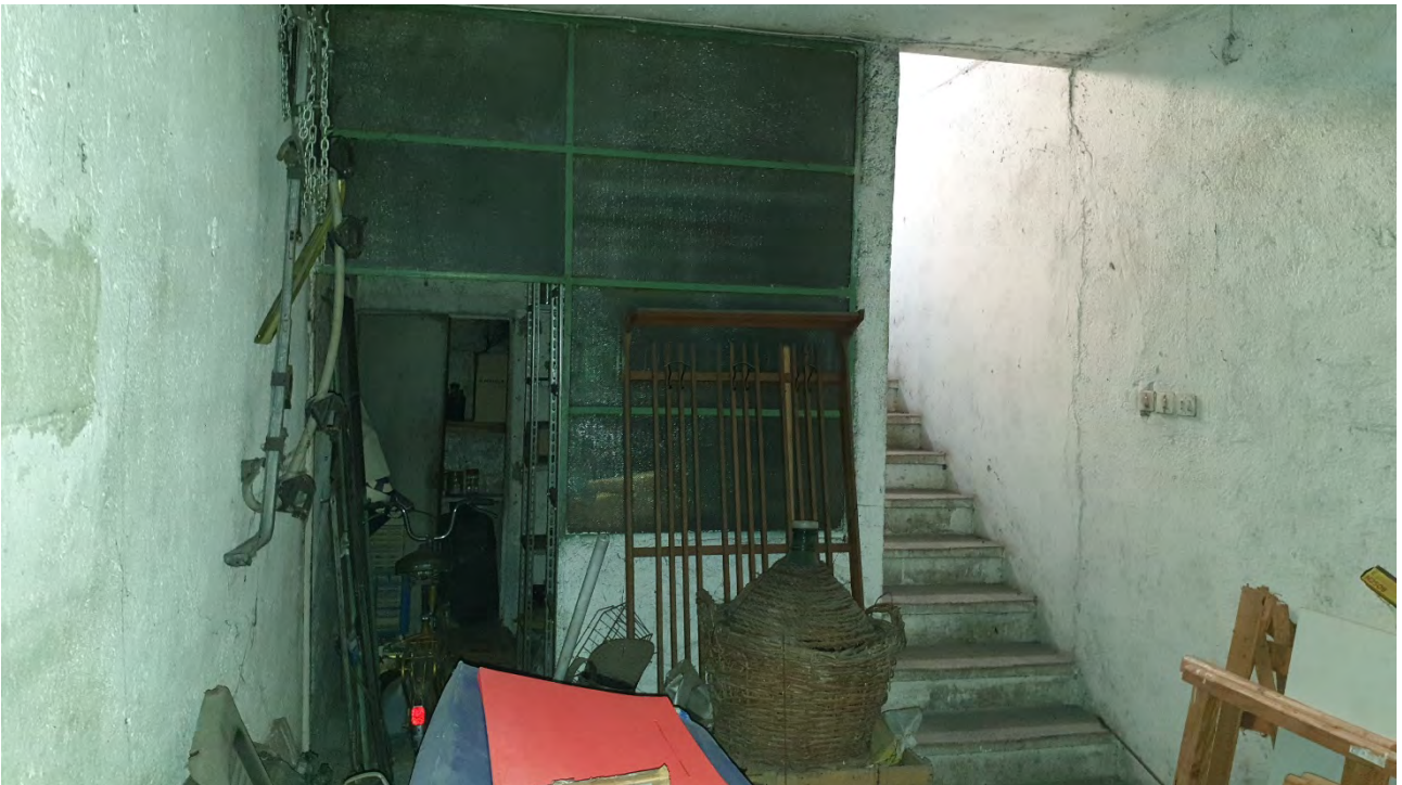
VISTA PIANO INTERRATO
